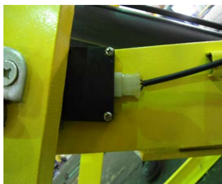
Picture 18 lower limit switch
